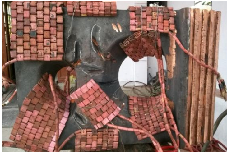
Fig.4 Heating position by resistors when welding and repairing
